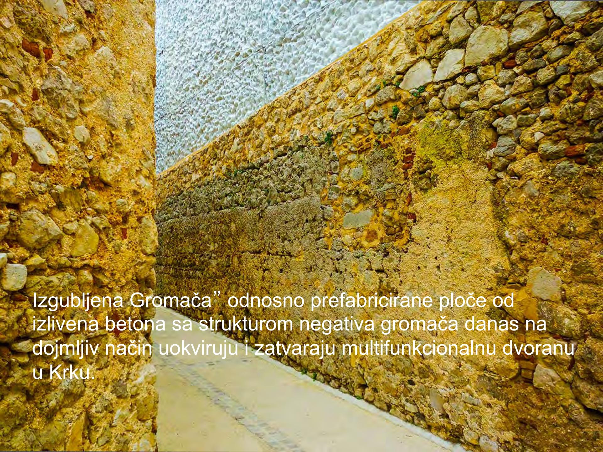
A photograph of a stone wall. On the left, there is a vertical section of the wall made of irregular stones. To the right, a large, light-colored concrete panel is attached to the wall, featuring a textured pattern of small squares. The concrete panel appears to be a prefabricated panel with a decorative gromača (stone block) texture.
